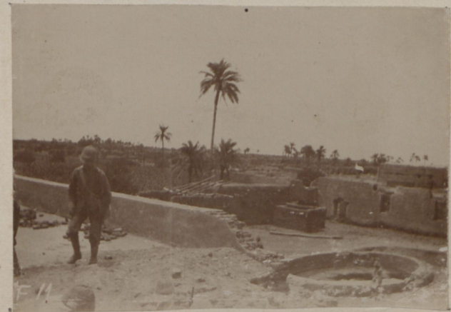
Khartoum 4 Sept. Courtyard from Roof
